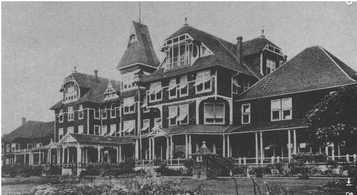
This photo shows Hotel Moldavia in Warren County, Indiana, where some Monroe residents went to get spa treatments in the early 1900s.
