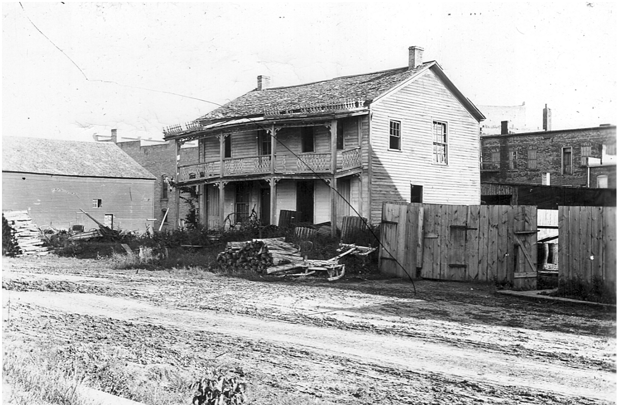
This photo of the Monroe House in its dilapidated condition was scanned from page 64 of the Monroe Area Pictorial History. The hotel was operated by Joseph Kelly on the north side of the square until it was moved to the opposite side of the block along 9th Street.
