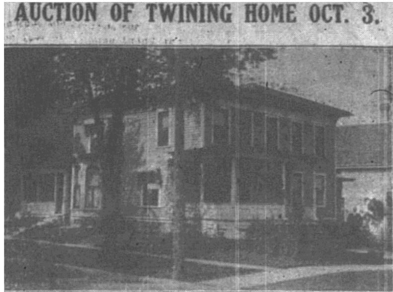
This photo of the Twining family house at 1423 15th Avenue was copied from The Monroe Evening Times of September 21, 1914 when it was “for sale.” There is a lot of history in this old house, part of which dates back to the 1860s.
