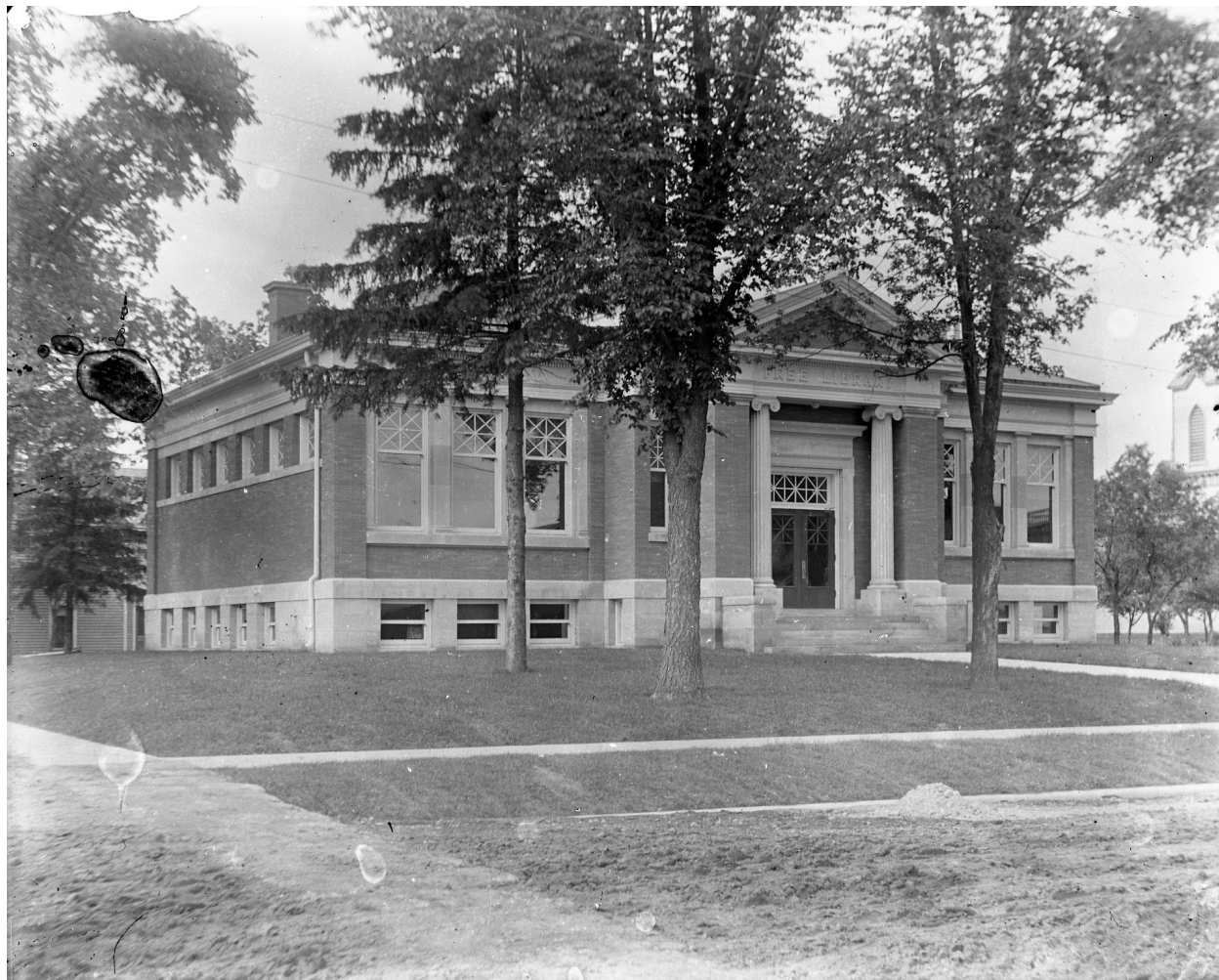
This photo, from the collection of the late Albert and Marion Deppler, shows the recently constructed Arabut Ludlow Memorial Library. Thanks to Edwin Ludlow and his brothers, this building was opened on May 22, 1905. The former Presbyterian Church (seen on the right) was razed in 1910.
